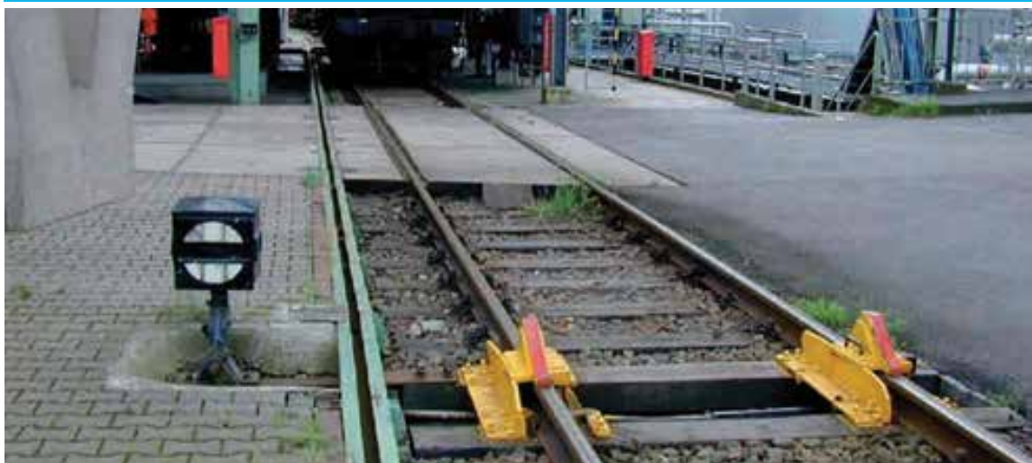
Fig. 6 Derailer at a filling station to prevent other railcars from entering the loading station
