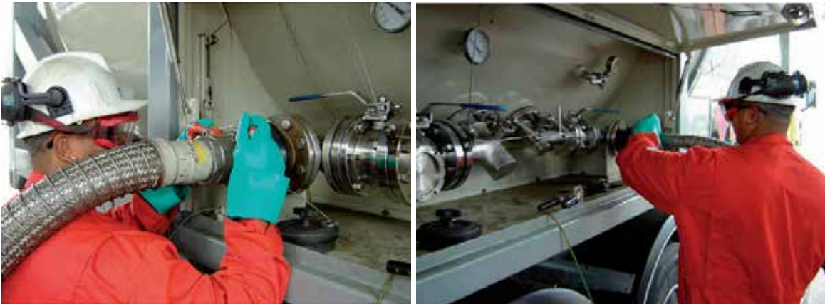
Fig. 4/5 Worker in protective clothing, connecting DDC liquid connection
