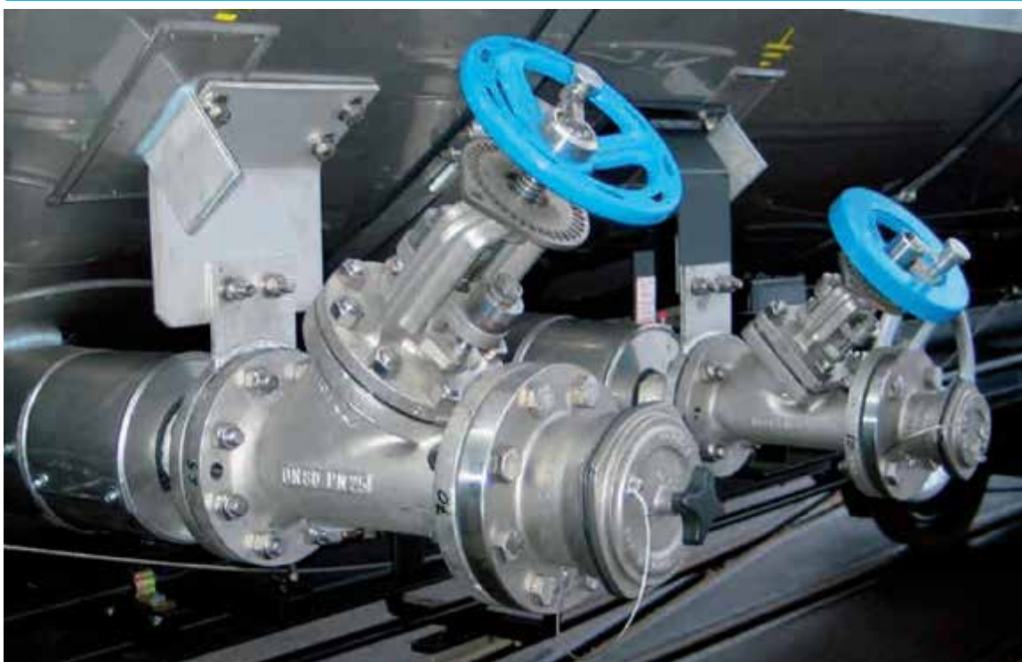
Fig. 2 Dry Disconnect Coupling connection
