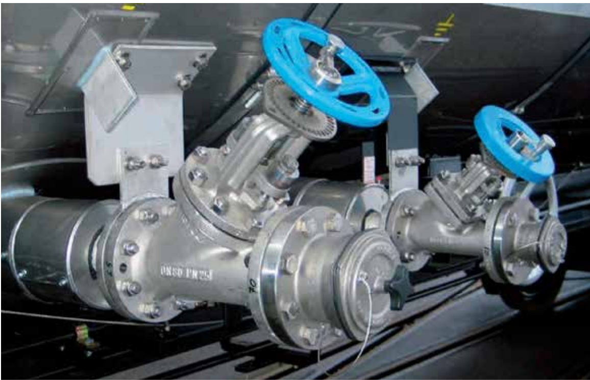
Fig. 2 Dry Disconnect Coupling connection
