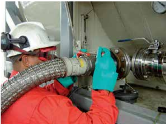
Fig. 4/5 Worker in protective clothing, connecting DDC liquid connection
