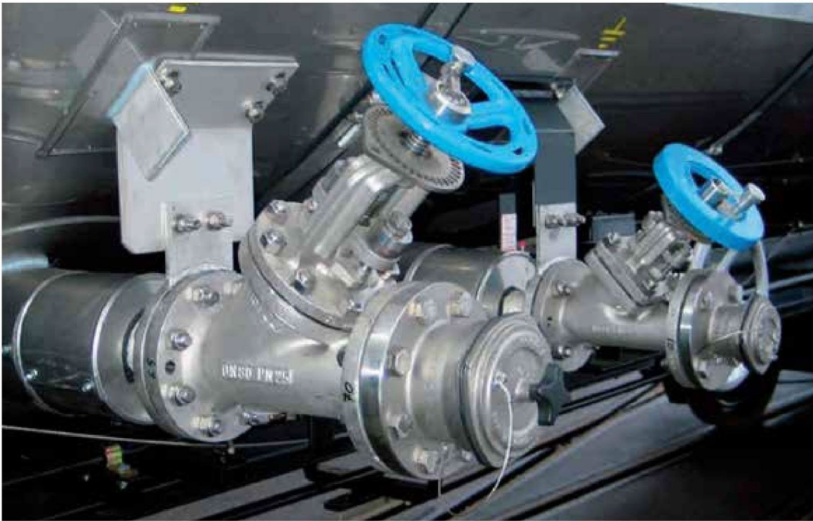
Fig. 2 Dry Disconnect Coupling connection
